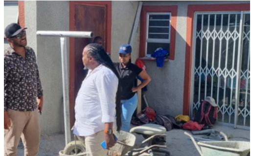
Above: Site visit by the DAG and Planact team to one of the sites worked on by a DAG-trained contractor.
