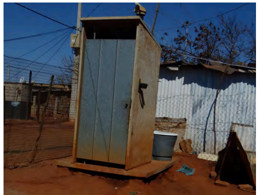
Above: A picture of a ventilated improved pit latrine (VIP) in Thembelihle, south of Johannesburg.
