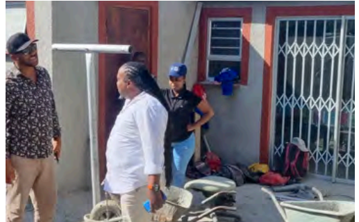
Above: Site visit by the DAG and Planact team to one of the sites worked on by a DAG- trained contractor.
